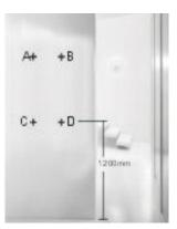
Drill a pilot hole into each marked point.
