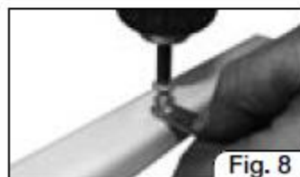
REMEMBER TO OFFSET SCREW FOR FLAT BRACKETS
