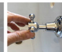
5. Insert the handle base into the headwork
