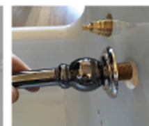
6. Screw the tap mouth into the central hole
