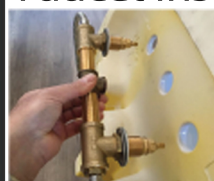
1. Insert the pipes in the holes
