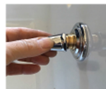
4. Screw the cap to the headwork
