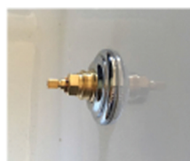
3. Screw the faucet stud on the headwork
