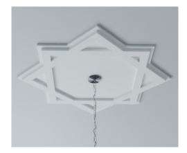
**CONSTRUCTION:** Expanded Cellular PVC
