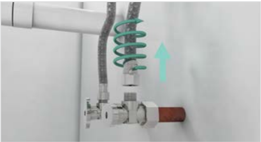
Diagram 2.3(B).5 Detach Cold Water Feed Line
