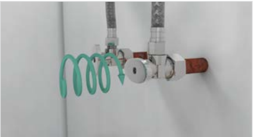
Diagram 2.3(B).4 Shutoff Cold Water Source Valve
