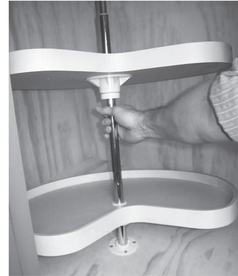
From the bottom of the pole, slide one Shelf Assembly, the Shelf Support, and then the other Shelf Assembly onto the Pole Assembly. Slide bottom of Pole Assembly into the Lower Mounting Bracket.
