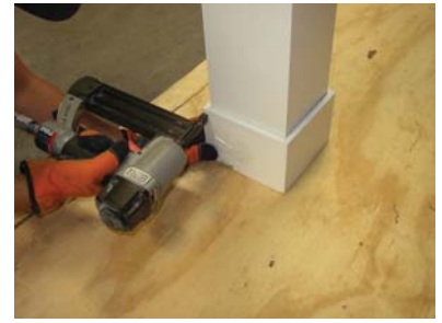
12) Fasten joints on base with pin-nails.
