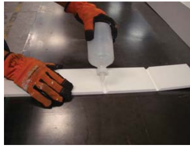
11) Apply adhesive to mitered edges of base moulding and wrap around bottom of column shaft.
