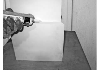
15) Caulk edges of base, cap, and nail holes.
