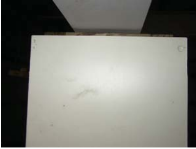
13) The TOP of the shaft should NOT be fastened to the post and there should be at least 1/2" gap to allow expansion (see step 2).
