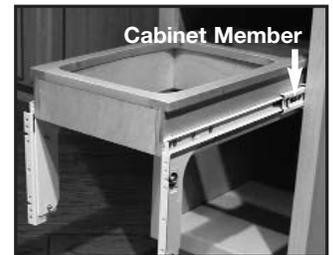
Step 5: Attach rear of cabinet members to spacer blocks. Center of cabinet members should be 14 1/4" from cabinet floor (center of spacer blocks).
