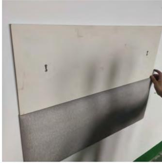
**12** Once the second position has been marked, drill 1/4 of inch for anchor placement, insert the anchors, drill in the screws and install the template. You may refer to step #8
