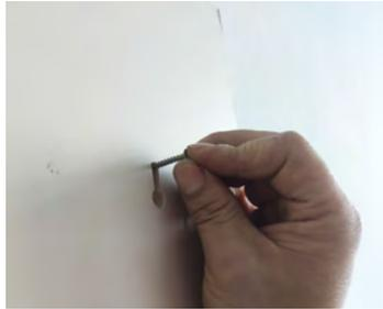
**2** Place the template and mark the location with the use of screws.
