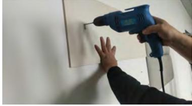
**11** Place the template on top of the installed panel and mark the position
