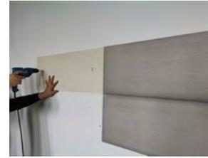
**14** Press the template firmly next to the installed leather panel and mark the location (See step #2)
