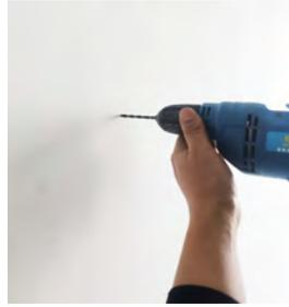
**3** Drill the holes for anchor placement (1/4 mesh)
