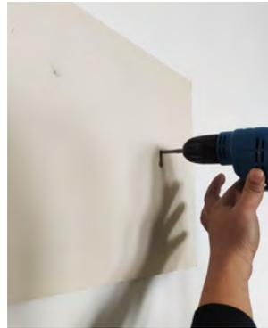
**8** Tighten the screws so that the template is pressed against the wall but has enough space to move up and down
