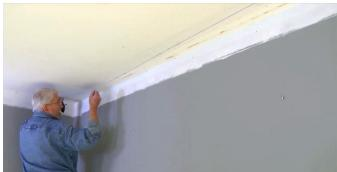
Measure the width of the border tile at each end from the wall. Drive a small nail at one mark and stretch a chalk line between the nails.
