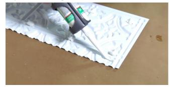
Use a high-tech, high-strength water-based adhesive suitable for ceiling tiles. Place nickel-sized dollops of adhesive in the field and run a small bead around the outside edges.
