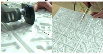
Begin laying perimeter tiles, starting from one corner of the room. Transfer measurements from the back of the tiles using a straight edge to draw a cut line.
