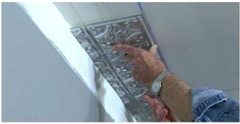
After installing perimeter tiles on two walls, begin putting up field tiles. Use the overlapping edge design for alignment.
