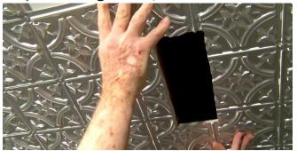
Measure from the edge of the nearest full tiles to the center of the electrical box. Mark the intersection of those dimensions, draw a circle, and cut out the opening.
