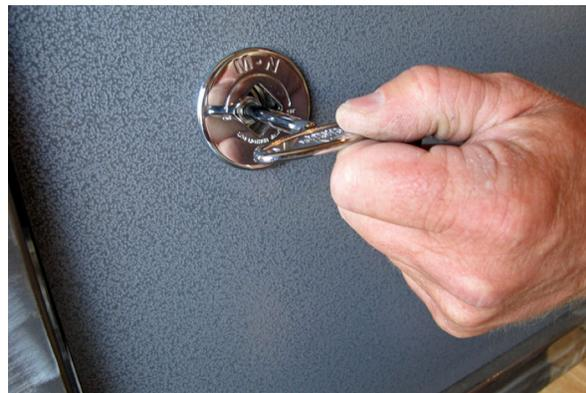
2. Turn the key valve clockwise toward the 'OFF' position until it no longer turns.
