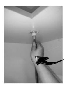
Holding onto the lower pole twist the upper pole counter clockwise to release. Extend pole upwards until it rests firmly against the Top Mounting Support and tighten by turning the pole clockwise.
