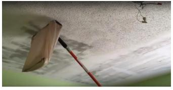
Styrofoam ceiling tiles can be installed on ceilings and walls covered with drywall, lime, lime-cement, dry plaster, chip-board, aerated concrete, masonry, silicates, and popcorned or textured ceiling finishes. When installing over any existing ceiling material, the surface should be dry, stable, even, hard, and free of any dust or debris.
