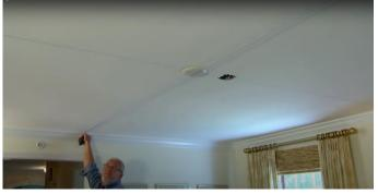
To achieve an aesthetically pleasing layout, it is recommended to begin installing your Styrofoam decorative tiles from the center of the room. If there is already a ceiling fan or light in this location, you can start there. Otherwise, you can use the string method to determine the room's center.
