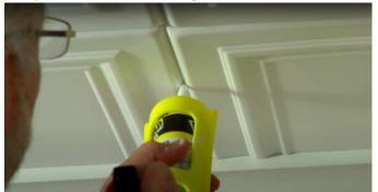
After completing the tile installation, use a caulking gun to apply caulk along the tile seams, focusing on areas with gaps for a seamless look. Practice caulking on spare tiles if you're inexperienced before working on the finished ceiling.
