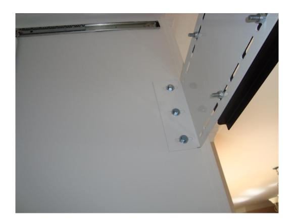
Once the bracket has been installed and all bolts tightened down you are ready for the wire management and TV installation. At this time please test the stability of the SlydLock mount to make sure you have hit studs and the mount will support your TV and the included weight.
