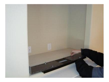
The adapter plates are secured with 8 Carriage bolts (Do not over tighten the carriage bolts, we will have to make a slight adjustment later) that can withstand the force of 400 lbs. Just secure the locking nuts on each bolt and you are ready. Make sure you install the bolts as pictured or the thread from the bolts will get in the way of the TV bracket! (Should be smooth side faced out with the bolts out the back of the mount)
