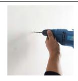
Drill the holes for anchor placement (1/4 mesh)
