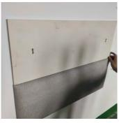
12 Once the second position has been marked, drill 1/4 of inch for anchor placement, insert the anchors, drill in the screws and install the template. You may refer to step #8
