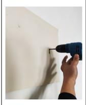
Tighten the screws so that the template is pressed against the wall but has enough space to move up and down
