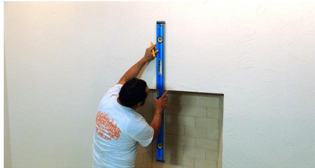
4. Find and mark the centers of all studs in the wall behind the *DeVinci Cast Stone* product and, using a level, transfer the mark up the wall to a point above the final height of the *DeVinci Cast Stone* product. These lines will identify attaching points during the build.
