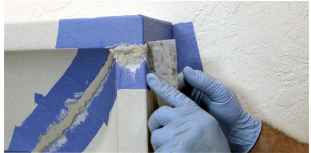
12. Once flush, the joints can be tooled smooth with a trowel, brushed with a horsehair masonry brush or rubbed with a piece of carpet.
