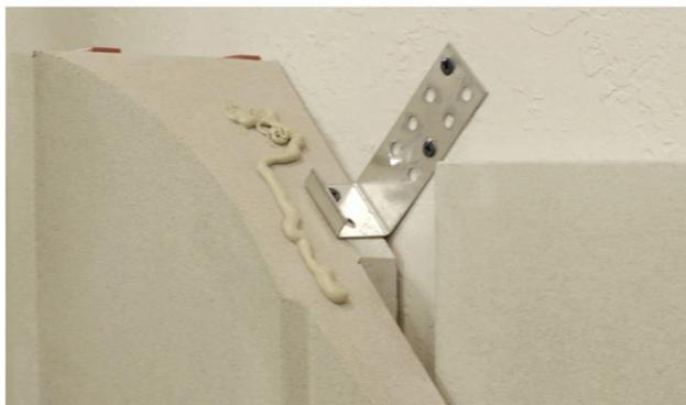
11. Put a small amount of mastic on the back surfaces of the mantle shelf / header that will meet the wall.
