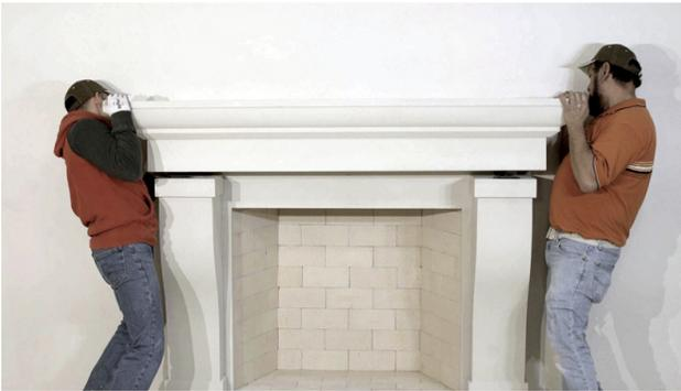
21. Check level side to side and front to back. Assure that top of header is even with top of legs.
