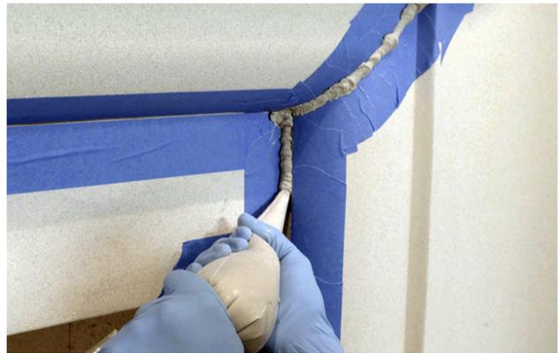
6. Fill grout joint liberally and work first course back into joint approximately  $\frac{1}{4}$ " to  $\frac{1}{2}$ " with tuck pointing trowel or similar tool.
