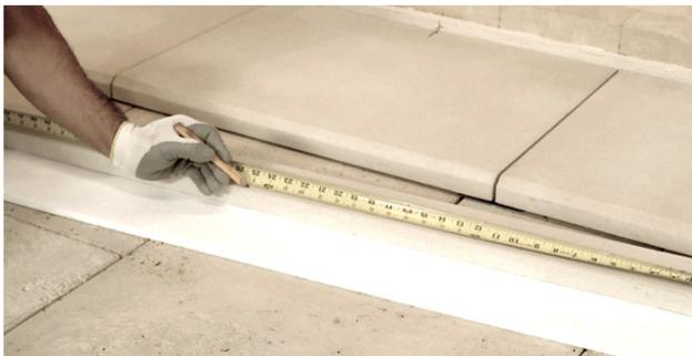
2. Position one-quarter inch of grout spacers on hearth or floor below outer edges of the fire box.
