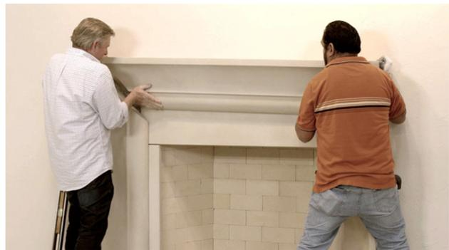
13. Check level side to side and front to back. Assure that top of header is even with top of legs.
