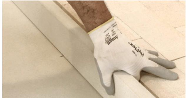
5. Check and adjust level as needed and secure the panel to the wall at its right and left outer edges using J-02 brackets.
