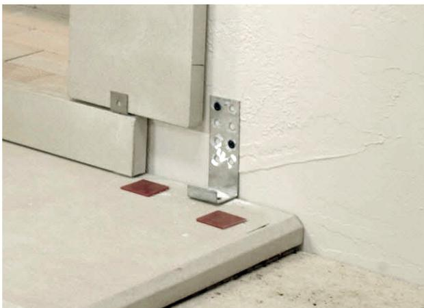
3. Place one-quarter inch of grout spacers on both sides of each J-01 Leg & Mantle mounting bracket.
