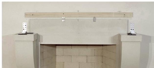
17. With the low edge of the chamfer on the top of the cleat (CL) facing the wall and its bottom edge centered on and aligned it with the horizontal line, Attach the cleat (CL) to the wall at three stud locations.
