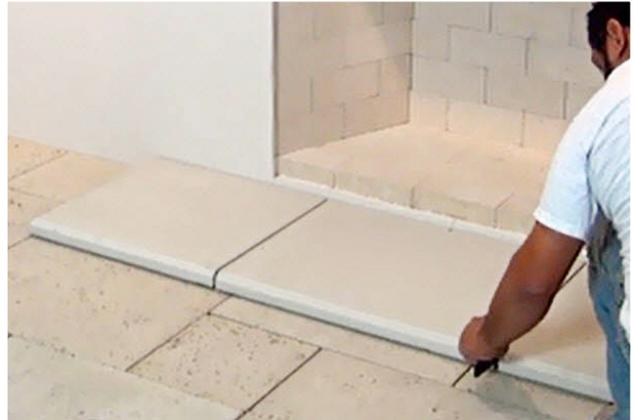
10. Compress mastic to level hearth stones side to side, front to back and appropriate height.
