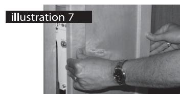
**Step 8:** Pull door open from sides of door at slide level. (See illustration 7). Make sure to securely tighten top screws.
