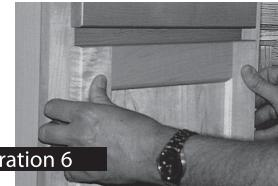
**Step 7:** Be sure bumper pads (not provided) are installed to all four corners of door. Push door closed and apply pressure to all four corners making sure door is flush with cabinet. (See illustration 6)
