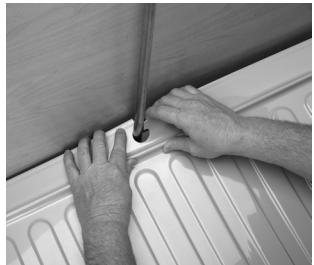
5) Use silicon adhesive around the entire perimeter and any holes you made for plumbing. Take care to seal all the cuts to ensure a water tight seal.
