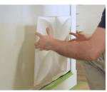
4.when the glue on the panel and wall is open air drying and sticky to fingers,install the 3d panel to the wall
