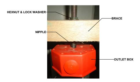
(Brace is above and not in contact with the outlet box and is accessible)
