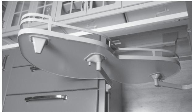
Position the lower swing arms outside the cabinet and install bottom tray into the pivots in each arm as shown above. Repeat for top tray and test motion of trays.
