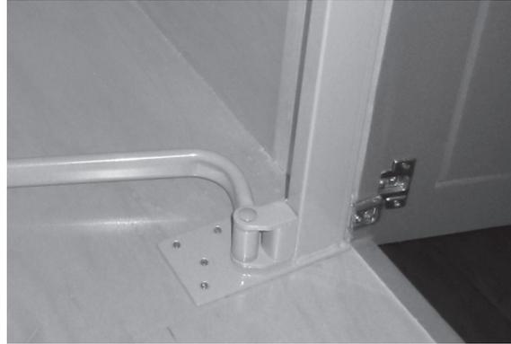
Firmly secure the Corner Support on the hinge side using (10) #6 x 3/4" flat head Philips wood screws.
