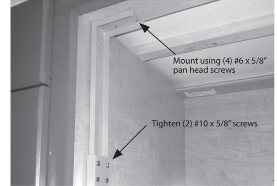
Lift the Telescopic Support Extensions until they are firmly against the bottom of the counter top or cabinet supports and tighten the (2) #10 x 5/8" washer head machine screws in the middle of the arms. Level arms and mark mounting locations. Then firmly secure using (4) #6 x 5/8" pan head wood screws in each top mounting frame bracket.
