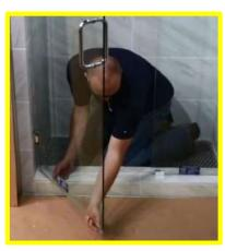
Press the drip over the bottom of the door with the angled water deflector to the interior
