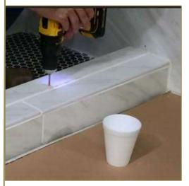
Drill the three marked holes. Cool the bit by placing in a cup of cool water every 10 to 15 seconds.
