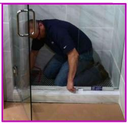
Use of the dam strip is optional but recommended if your curb does not have a slope to the interior. Measure and cut to length, clean the curb and apply with the double stick tape.
