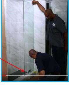
Use a tape measure to position the panel on the "backset" dimension and parallel to the outside of the curb.
