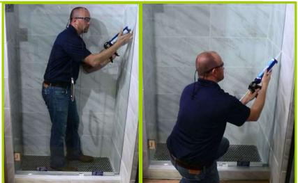
Do not use the door for 24 hours to allow the silicone to cure. Once the silicone has cured, Clean your new Symphony door with a soft cloth and glass cleaner. Be sure to remove the Enduroshield<sup>™</sup> labels from the glass and follow the instructions to register for the ten year warranty. Refer to the Enduroshield<sup>™</sup> website for more detailed cleaning instructions.
