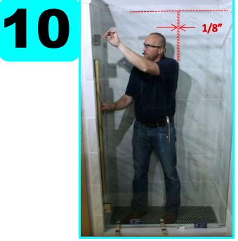
Carefully maintain the position of the door and double check it for plumb. Mark the six holes with a Sharpie<sup>™</sup>.
