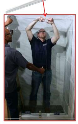
With your helper, carefully place the door into position on the spacers. Press the clear drip rail over the top of the door and panel to hold the door in position.
