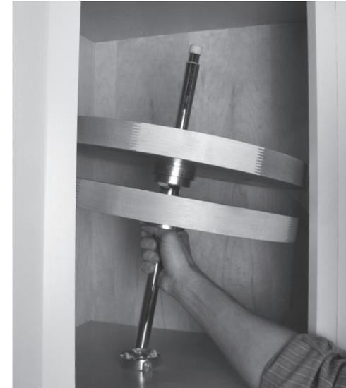
From the top slide one shelf, the other Shelf Support, and then the other shelf onto the Pole Assembly. Slide bottom of Pole Assembly into the Bottom Mounting Support.
