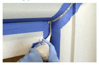
6. Fill grout joint liberally and work first course back into joint approximately ¼" to ½" with tuck pointing trowel or similar tool.
