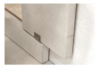
9. Check and adjust level as needed and secure the panel to the wall at its top edge using a J-02 bracket.
