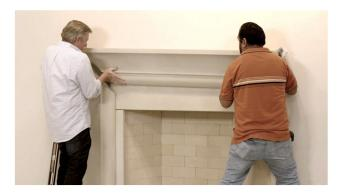
13. Check level side to side and front to back. Assure that top of header is even with top of legs.
