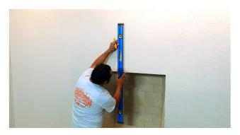
4. Find and mark the centers of all studs in the wall behind the *DeVinci Cast Stone* product and, using a level, transfer the mark up the wall to a point above the final height of the *DeVinci Cast Stone* product. These lines will identify attaching points during the build.
