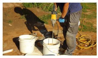
c. After initial mixing is complete, allow grout to rest for approximately five minutes and then re-agitate. This will break the grout's initial bond and make it easier to work in the grout bags.
