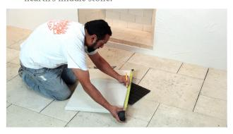
6. Shim mounting surface as necessary to gain appropriate base height and level side to side and front to back.
