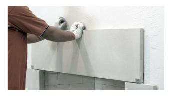
16. Check and adjust level as needed and secure the panel to the wall at its top edge using two Z-01 brackets.
