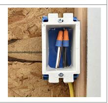
Using one of the in-wall junction boxes described above, there are two methods to supply power to a Docking Drawer or Style Drawer outlet.
