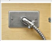
Single gang cover plate with a Flex 90 connector using MC to connect to the Style Drawers handy box
