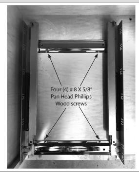
Place the slide base inside the cabinet, pulling the front cross member tight against the rear of the face frame. For frameless cabinets, set the front cross member back 3/4". For inset door applications, slide the base back from the above measurements plus the thickness of the door. Firmly secure with four (4) # 8 X 5/8" Pan Head Phillips Wood screws provided in the locations shown above.
