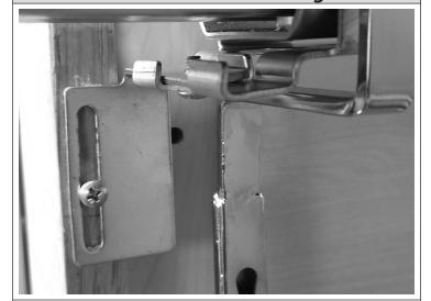
Pull the top front mounting bracket into position on the side of the face frame (or cabinet) allowing for a 3/16" setback (shown left above). Firmly secure with one (1) #8 x 5/8" Pan Head Wood Screw. Make sure the gap between the unit and the side of the face frame is equal from top to bottom. Adjust accordingly and then securely tighten the bracket set screw (shown right above). Operate the unit and make adjustments as necessary for the slides to operate smoothly.
