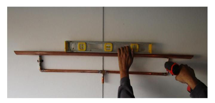
2. Measure down 25 ½" from the center of the bottom of the disperser pipe and make a mark
