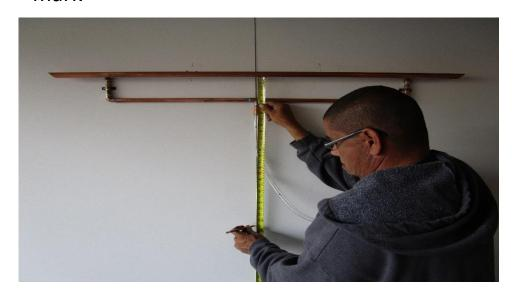
3. Install pan bracket to wall making sure the top of the bracket is on the mark made in step 2, insure bracket is level.
