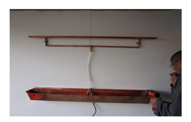
6. Using a level or other sturdy flat item and place across the base pan. Place slate panel on level (or flat surface). Fold copper straps over disperser pipe and attach with provided hardware.
