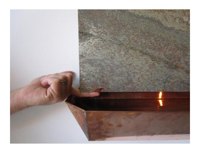
8. Fill base pan with water, do not over fill. Plug in pump and make sure water flows evenly. Use a wet sponge to insure the entire slate panel is wet.
