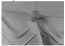
Secure the panels by applying pressure on flat surfaces of panel. Allow 24hrs interval before painting if required.
