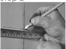
Pre-mark wall according to product dimension to ensure straight and level installation Step 5
