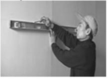
Ensure wall surface is clean and dry prior to installation. May require roughening of wall surface by sandpaper for better grip.
