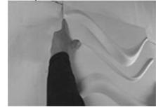
Align pieces according to pre-marked lines and ensure pieces are tightly butt next to each other.
