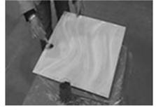
Apply max bond construction Adhesive evenly on back surface.
